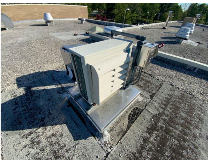
17 - SPLIT SYSTEM DUCTLESS
